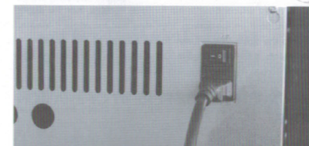
Figure 20a: Main power switch
